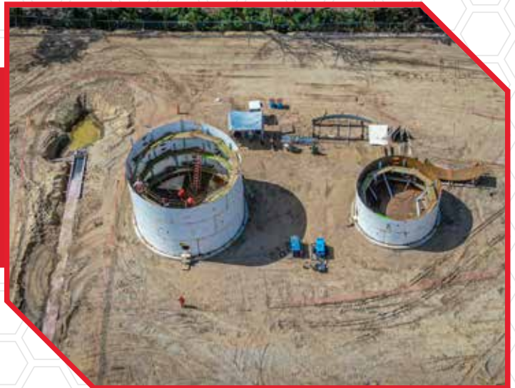
Water storage tanks over improved soil.
