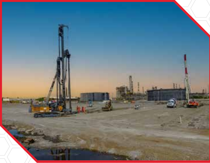
Execution of CMC in refinery.
